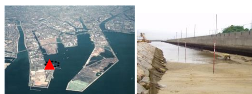
Fig. 1 The artificial tidal flat of Amagasaki port in Osaka bay (Length 32m, Width 12m, Highest tide level:O.P.+2.1m, Lowest tide level:O.P.+0.5m(O.P. : Osaka peil), Slope:2%(1/50), Sediment : Sandy
